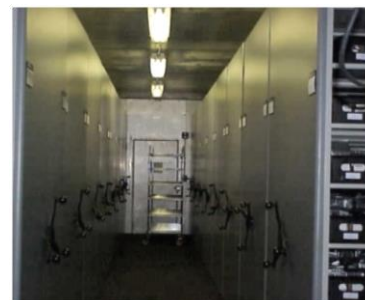
Freezer at -18 °C where most seed is stored to maximize seed longevity
